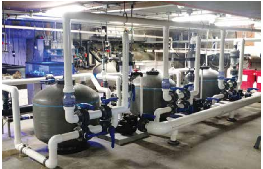
▲ Micron Side Mount fibreglass filters filled with Glass Pearl filter media and MultiCyclone centrifugal pre-filters.
