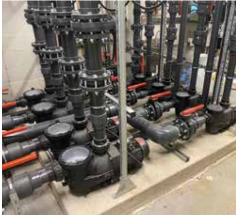
The 25m metre, 240 m 3 swimming pool relies on Waterco's proprietary fibreglass filters, Hydrostar commercial-grade pumps, and water-saving MultiCyclone centrifugal filters to maintain premium water quality.
