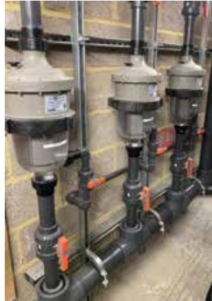
The 25m metre, 240 m 3 swimming pool relies on Waterco's proprietary fibreglass filters, Hydrostar commercial-grade pumps, and water-saving MultiCyclone centrifugal filters to maintain premium water quality.
