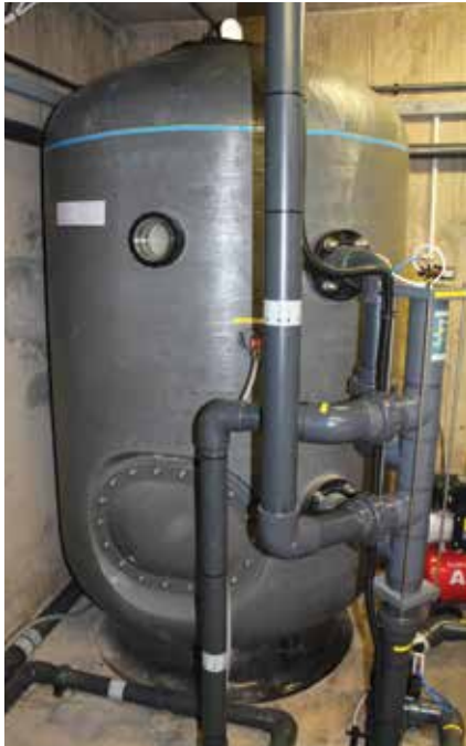
Waterco's fully automated SPDD1200 Nozzle Plate Filter with a 1.2m bed depth with Waterco Glass Pearl Media.
