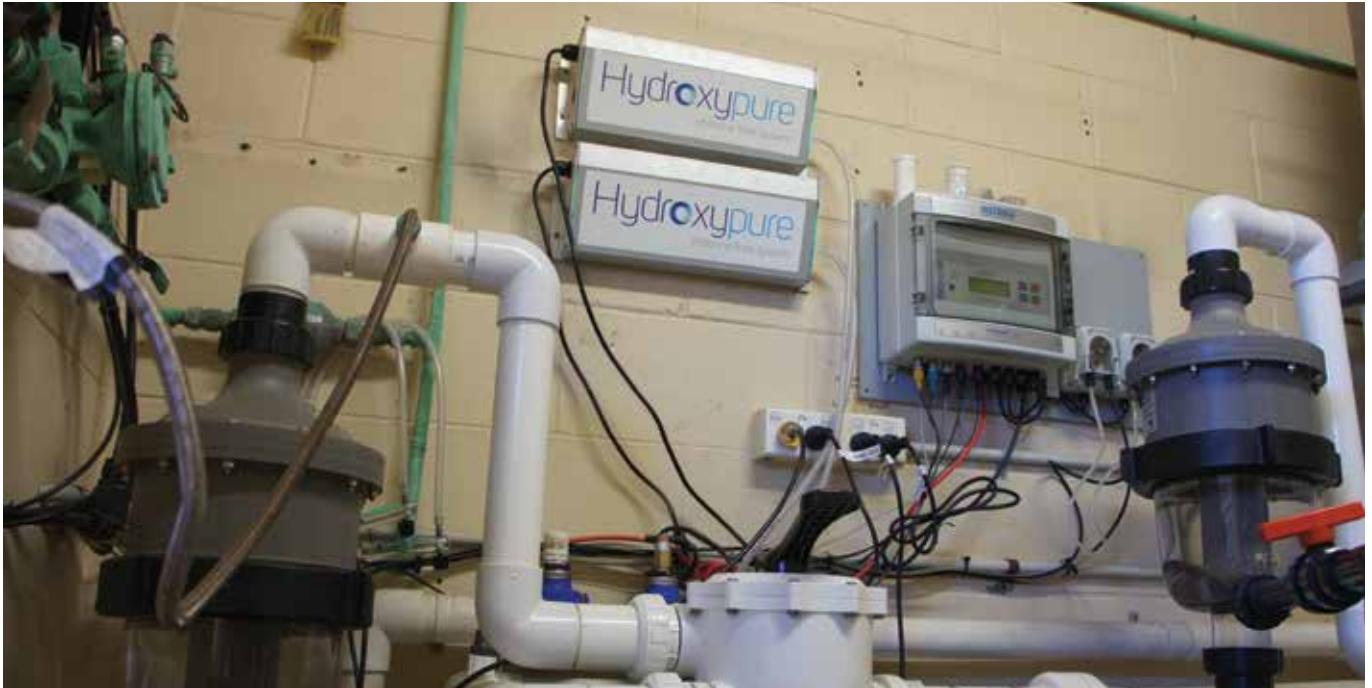
The Hydroxypure system is compact and easily retrofitted to the pool's existing plumbing system.
