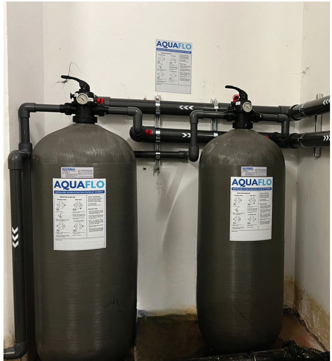
AquaFlo Filtration System in Action: The AQ600X units at Mercure Hotel, designed to improve water quality and reduce internal equipment strain
