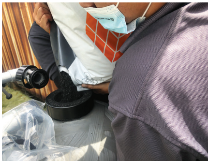
Waterco technician filling GAC-Plus into a W400 filter.
