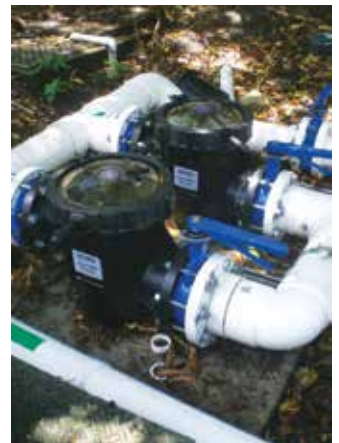
Two manifold Waterco Hydro5000 commercial strainers, which each feature a 150mm inlet/outlet and 16-litre strainer baskets.
