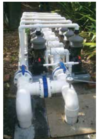
Ten manifold MultiCyclones focus on collecting the finer particles, where the flow rate through each ranges between 200-300-litres per minute.
