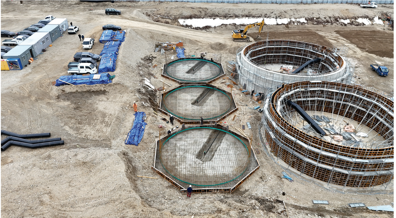
Early construction phase of the 28,000m 2 Test Bed, featuring reinforced tank structures. The biggest tank diameter is 21 meter with 6.5 meter height.
